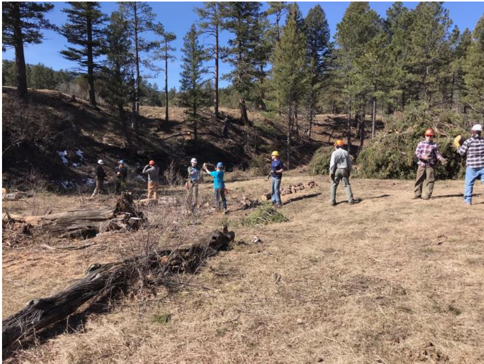
“The “log line” passing logs from the work site uphill to the road.”
